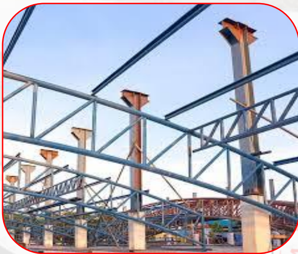
Structural for Buildings and infrastructure
